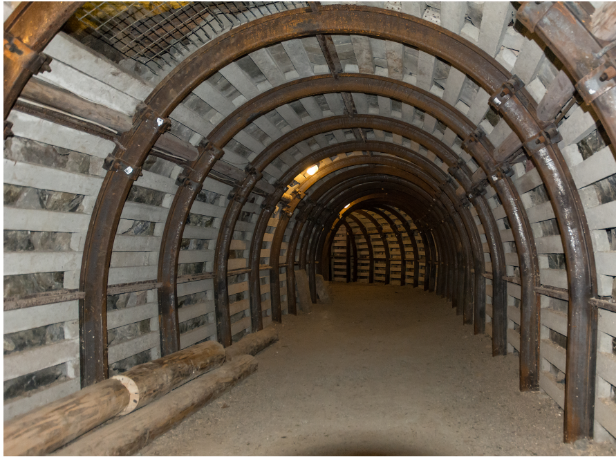
Fig. 5: View of steel arch yielding support ( https://upload.wikimedia.org )
